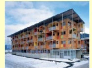
Low-rise wood structure
