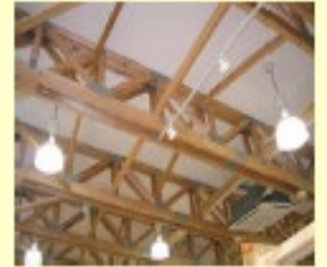
Parallel cord wood truss
